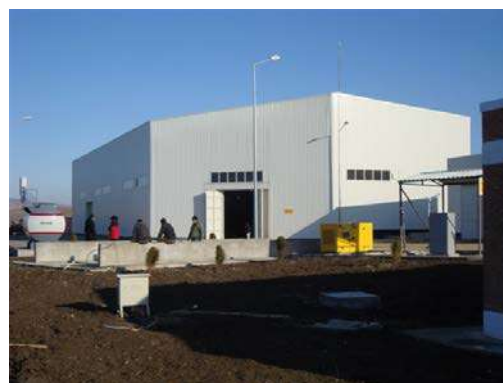
Waste Sorting Building
