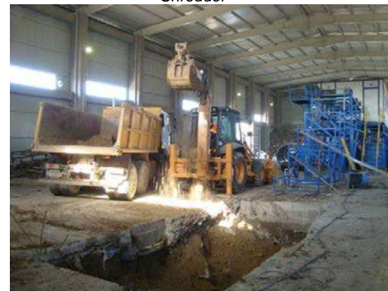
Re-construction of WSL
